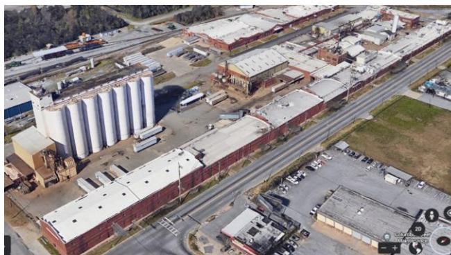
Fig. 3.1.9 FPU Location with Clean Surroundings
