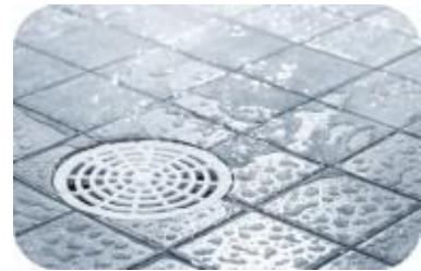
Figure 2.1.39 Cleaning the Drains
